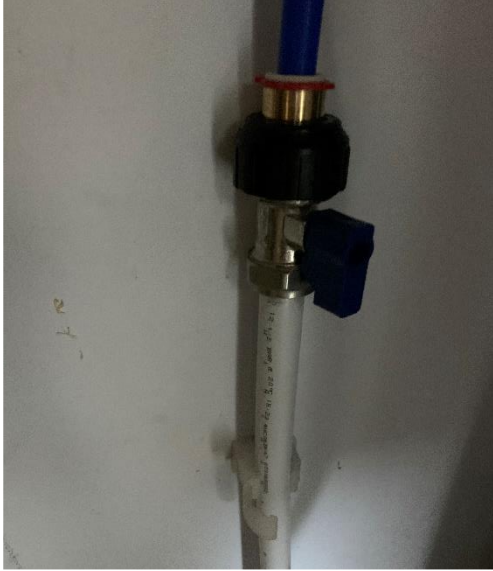
Picture above of what a valve looks like once connected to a coffee machine pipe.
